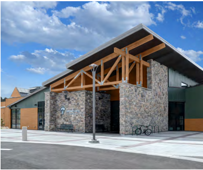
Estes Valley Community Recreation Center
