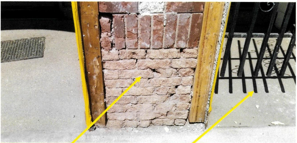
Typical brick replacement at column bases.
