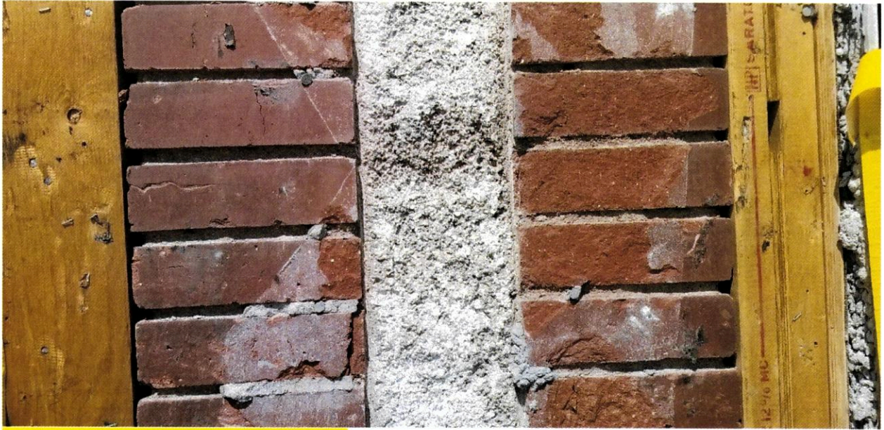
Typical brick replacement at columns.
