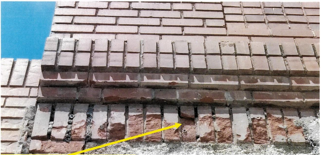
Typical brick replacement behind stucco.
