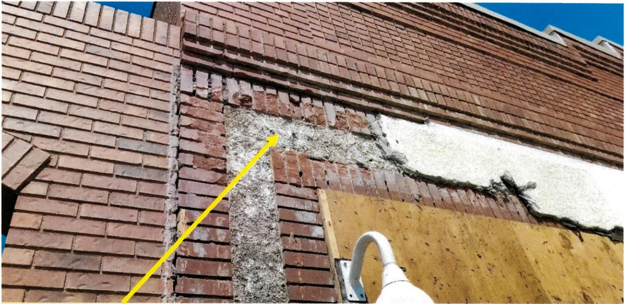
Typical historic stucco repairs.
