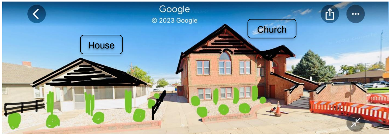
Figure 2: Street view of 2 properties currently on Block 15, 16, 17 and 18 of Twomblys
