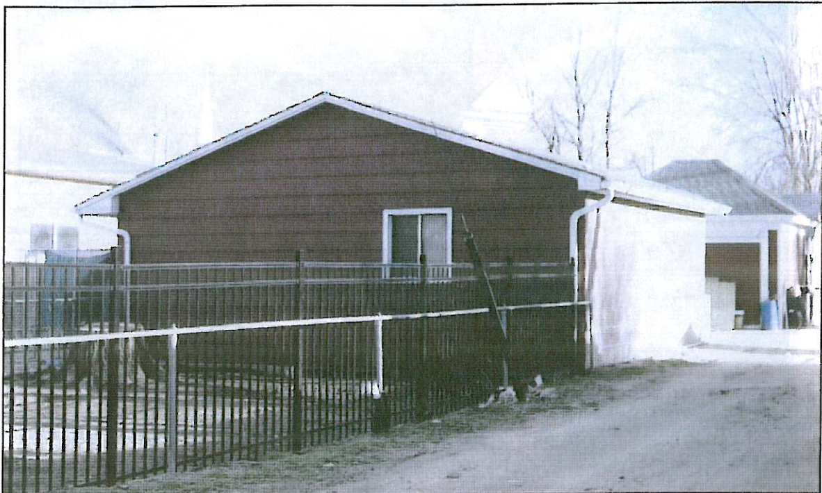
View of the new garage along the rear alley. View to the southeast.
