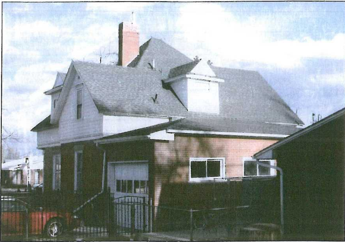
View of the north and west elevations. View to the southeast.
