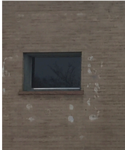
Old epoxy, and discoloration of bricks
