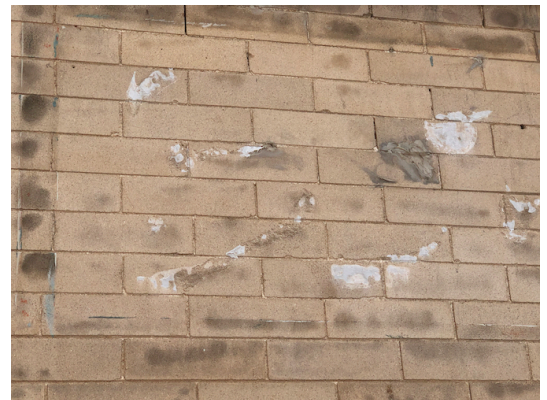
Old epoxy, and discoloration of bricks
