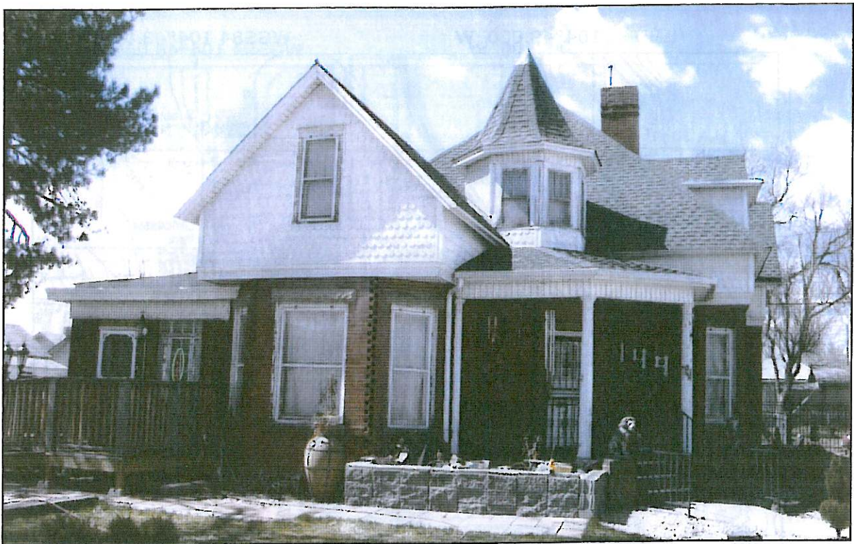
View of the east elevation of the Rhode House. View to the west.
