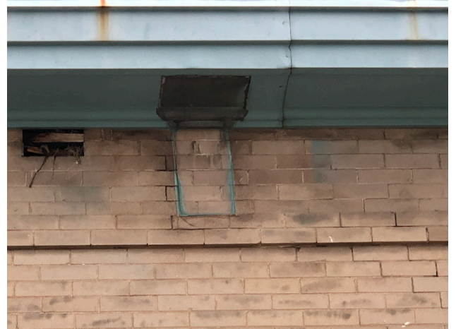
Cornice & Corbel repair and replacement
