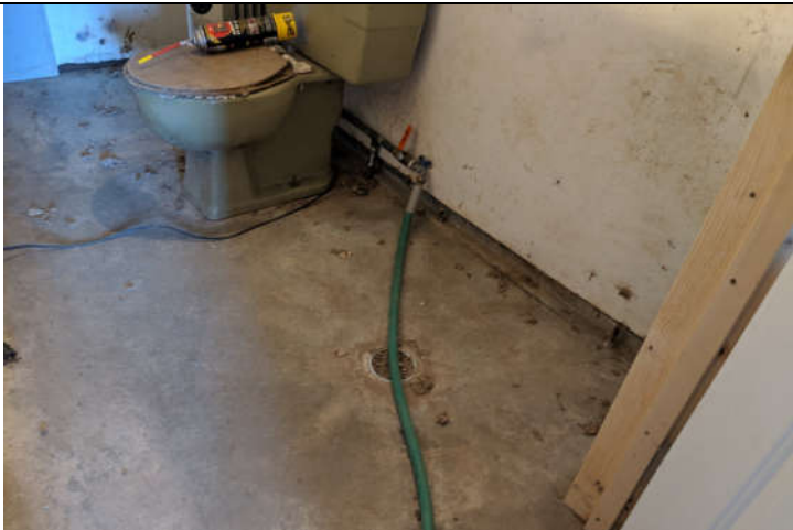
Description: Floor drain in bathroom of northwest corner of Quonset. Direction: Overhead/Northwest
