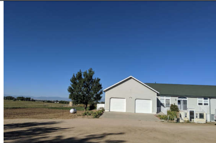
Description: West residence, leach field, and propane tank. Direction: West
