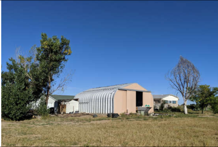
Description: Quonset hut, shed and disposal bin. Direction: West-northwest
