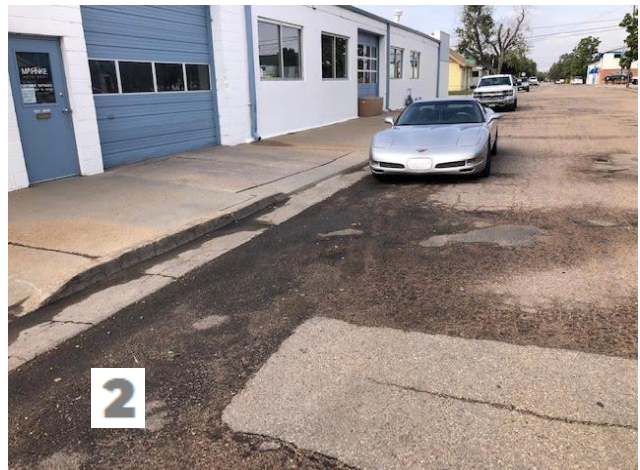
3. Close up of alligating, cracks, and disrepair on Sixth Street.
