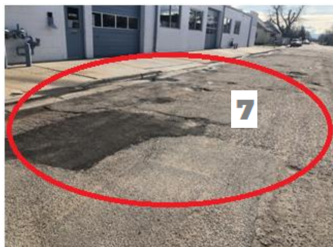
7. This picture shows the majority of the patchwork the contractor completed on Sixth Street, facing west.
