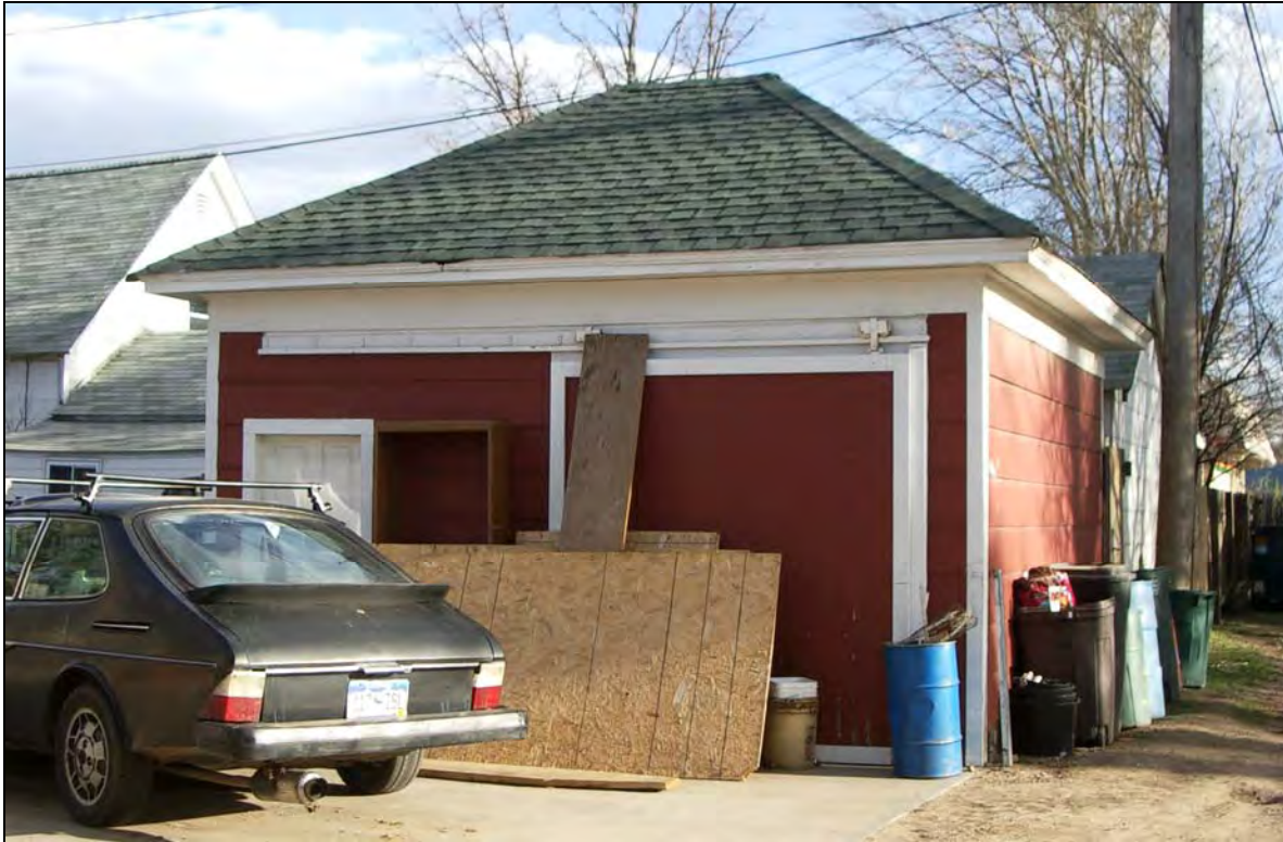
View of the old garage along the rear alley. View to the southeast
