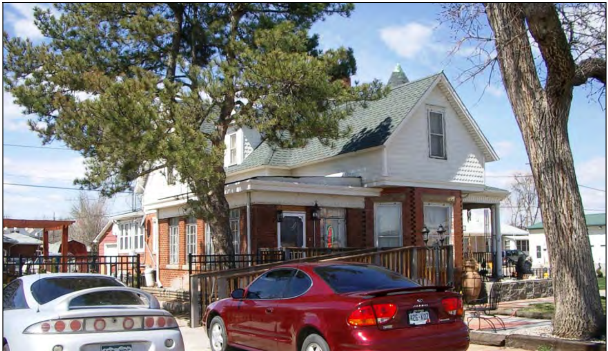
View of the south and east elevations. View to the northwest.
