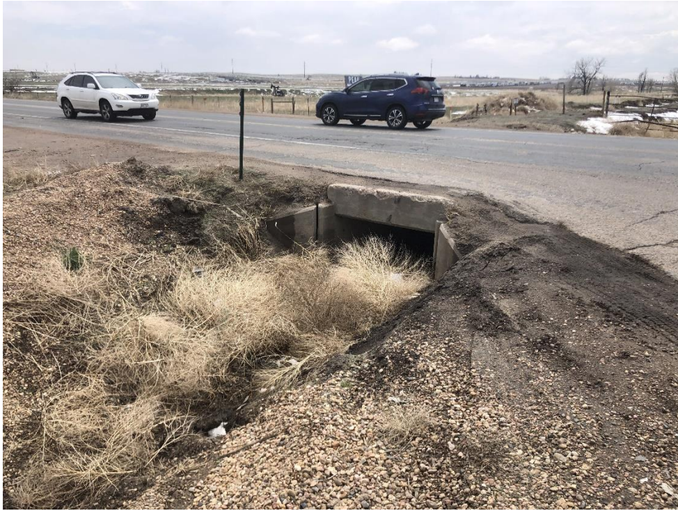
Looking toward State Highway (SH) 52 from Weld County Road (WCR) 19 – CBC (052A016420BR) - crossing the Brantner Ditch Segment (5WL.2649/5WL.2649.10)
