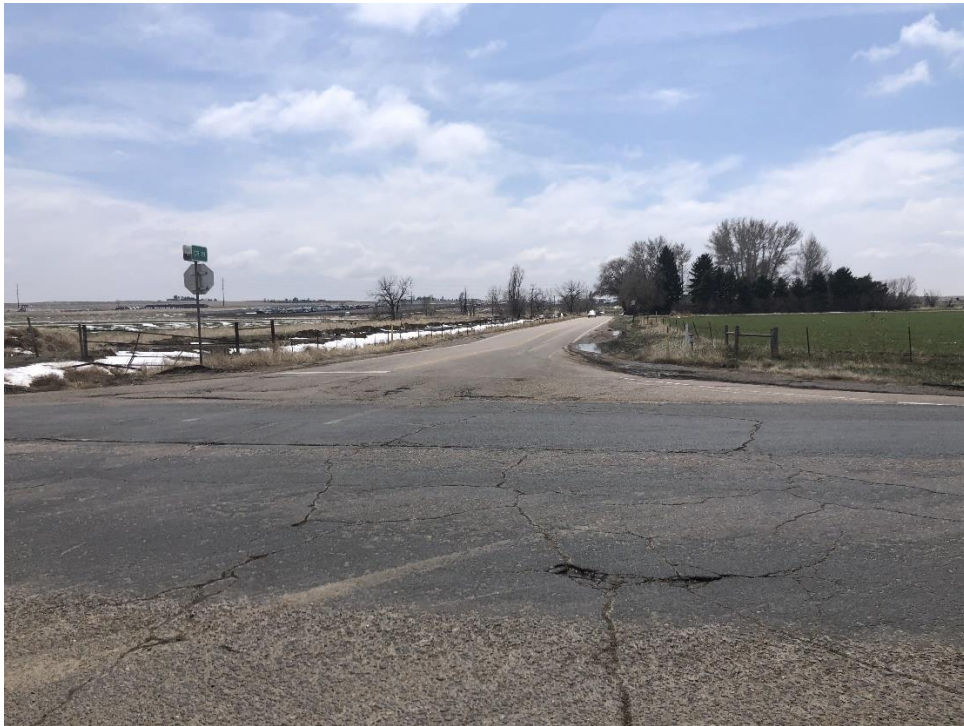
Intersection of SH 52 and WCR 19
