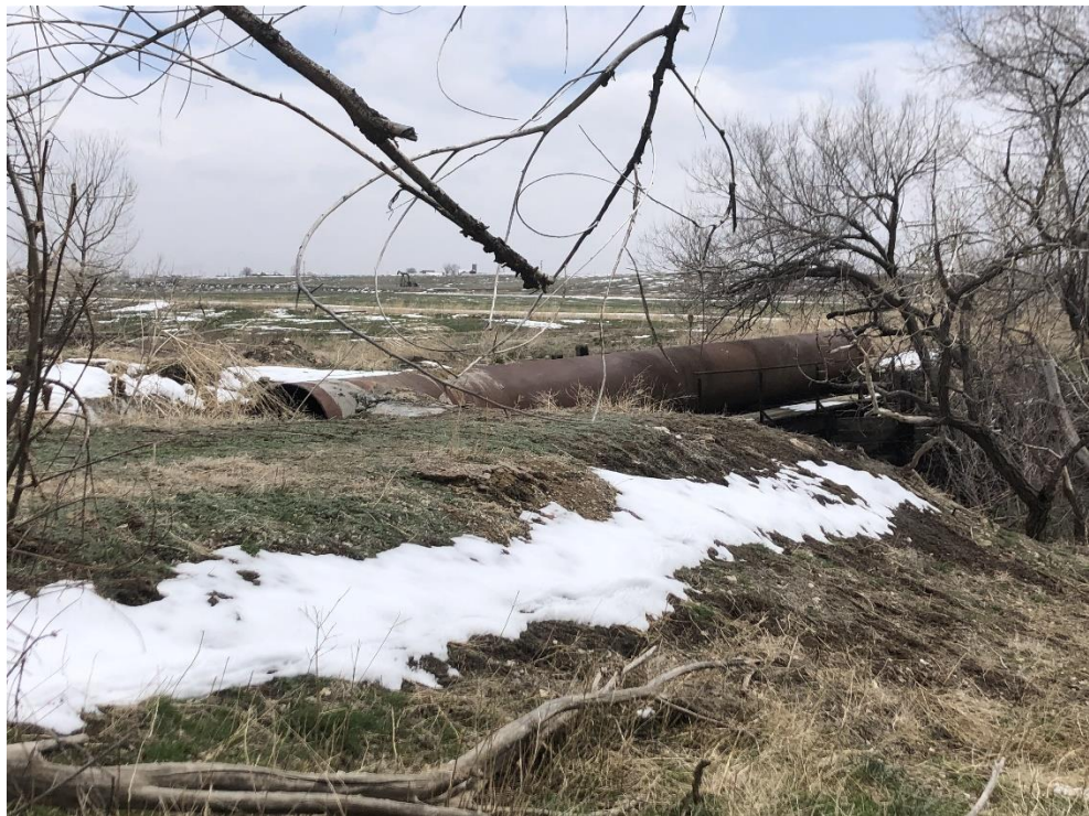
Piped Brantner Ditch Segment (5WL.2649/5WL.2649.10)
