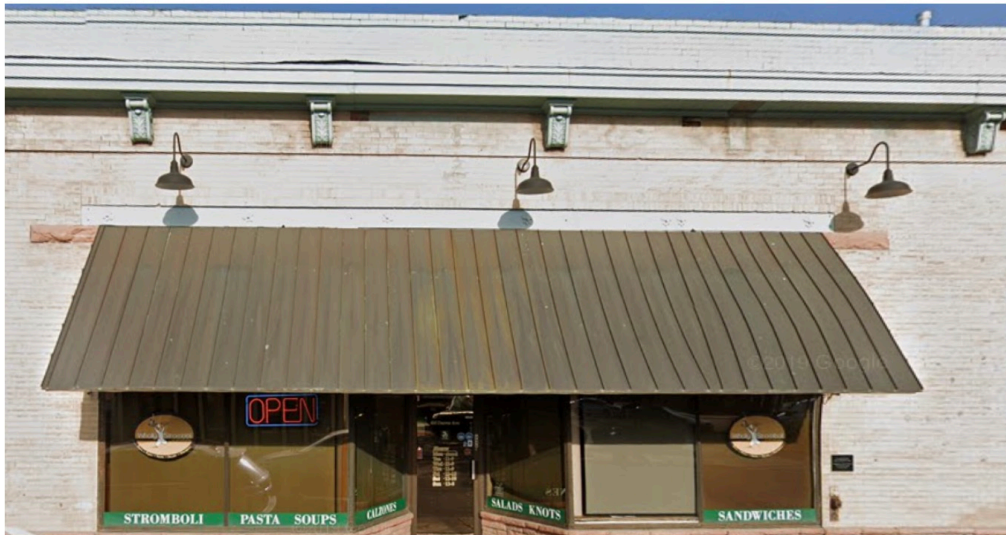
Photo depicting the Denver Ave facade - Existing Restaurant storefront
