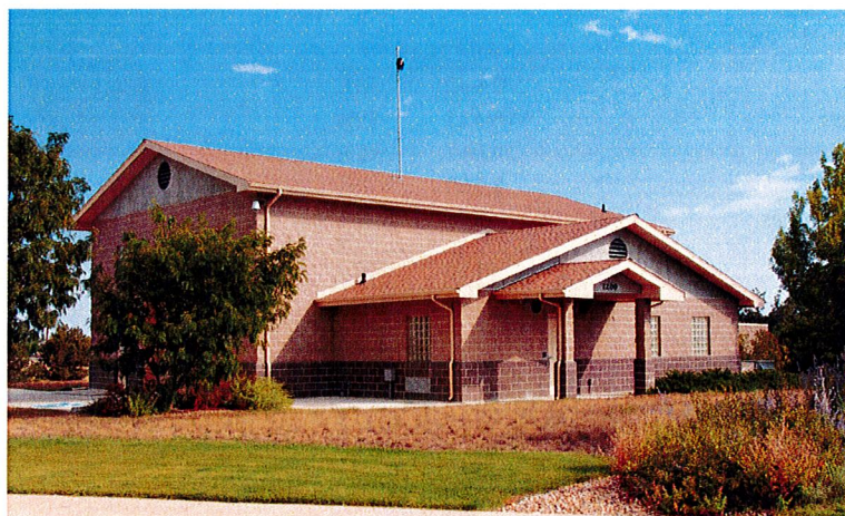
West Longmont Pump Station
